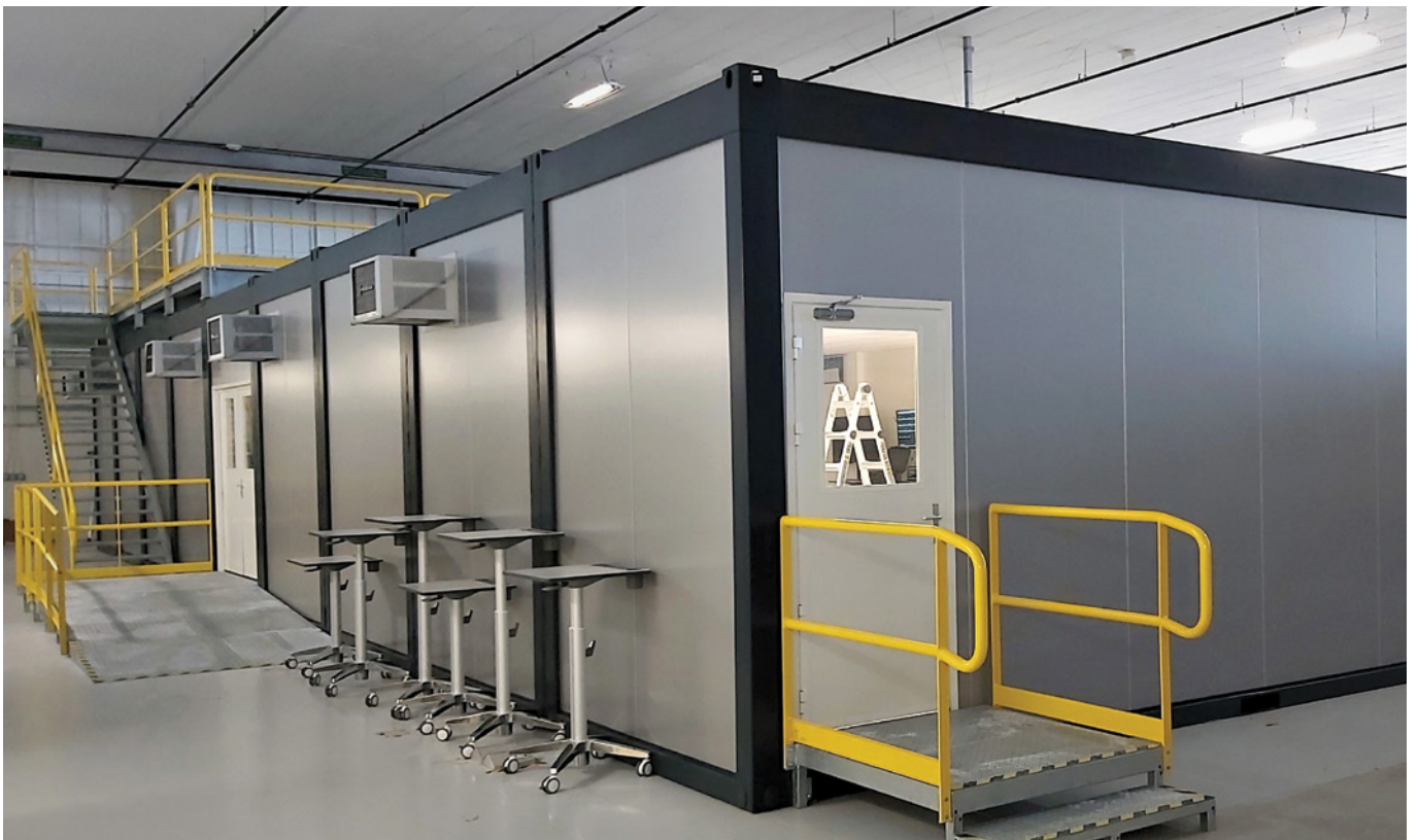
Flight simulator and office buildings with mezzanine at Randolph AFB
