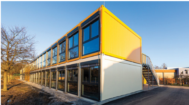
Offices made with OptiMax modules
