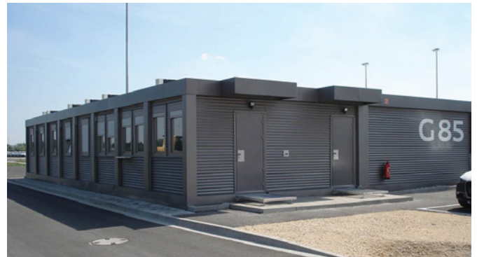
Private modular offices
